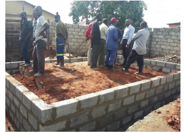
Construction of modern toilets in Lusaka
